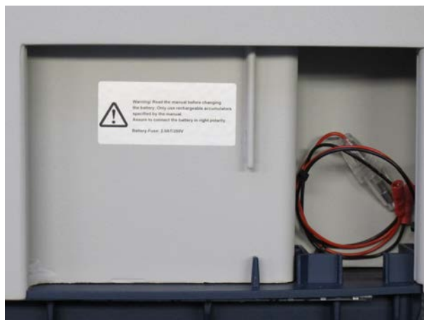
Figure 8.1: Accumulator bay with fuse
