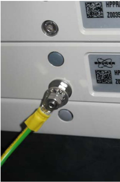
Figure 6.4: Connected Protective Ground Cable
