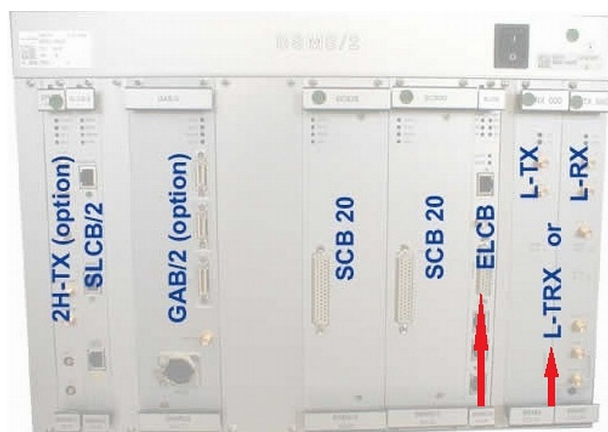
Figure 1.2: BSMS2 with ELCB board, L-TX/L-RX Boards or L-TRX Board
